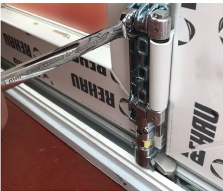
3: Adjust A + B nuts for horizontal movement
