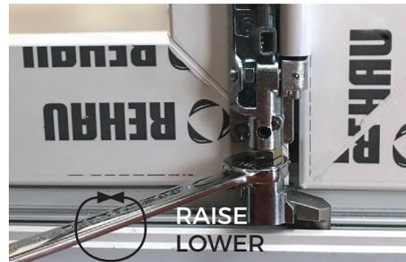
2: Turn nut to raise or lower sash with 18mm spanner
