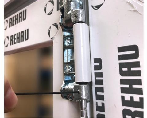
1: Slacken grub screws to remove pins - sash will come off
