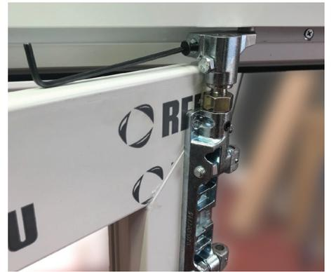
2: Removal of wheels - remove allen bolt
