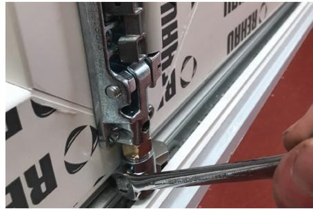
1: Slacken bottom nut on top and bottom rollers and move door for correct compression adjustment
