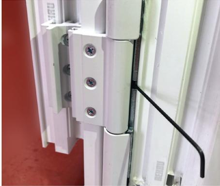
1: Remove grub screw with 2mm allen key
