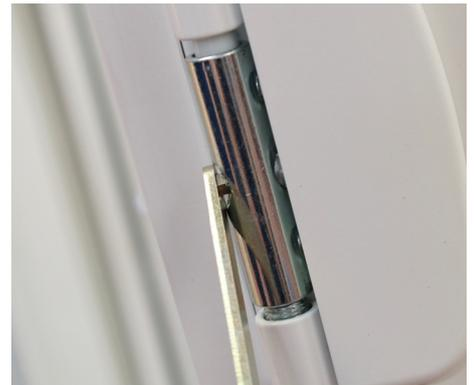
2: Adjust hinge using the hexagonal main hinge adjustment tool
